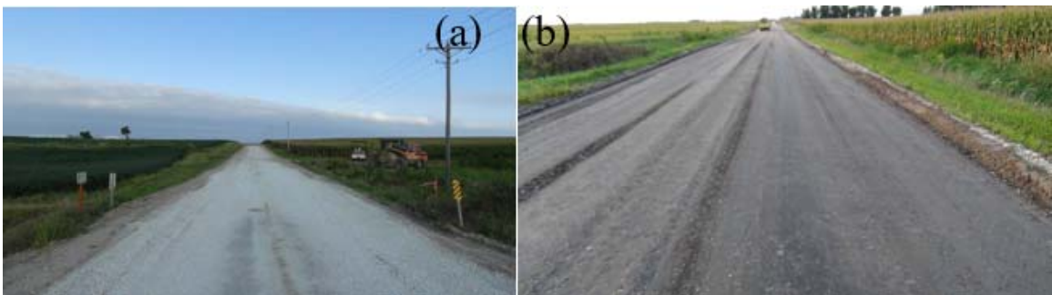
Figure 82 EMC Squared sections at end of construction (a) Washington (b) Hamilton
