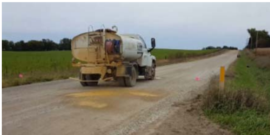
Figure 21 Tanker used for spraying clay slurry in Cherokee County
